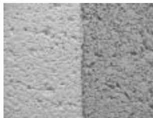
Other - CMU/Concrete Block Painted and Unpainted
